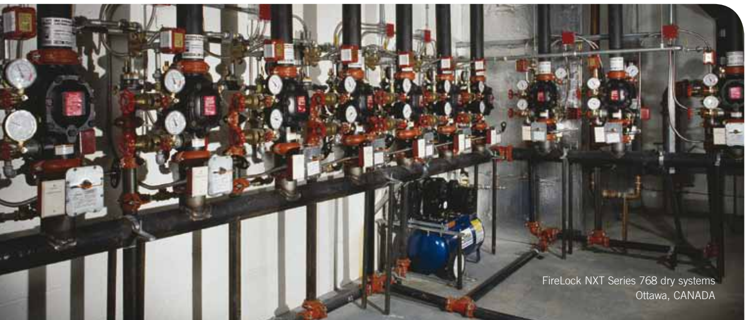
FireLock NXT Series 768 dry valve shown
